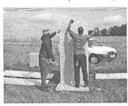
Place the second side panel in the recess onto the base slab (1st photo below) then push the two 945 rods through the side panel holes. Take 2 x M5 Nuts out of your accessory bag and turn it onto the two rods. Fasten the nuts tight with the spanners.
