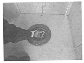
Push the three M8 x 90 set screws through the flange and base slab. Once the screws have gone through the holes, turn the M8 Nuts onto the screws and tighten with the spanner provided.
