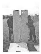
The sequence of placing the panels onto the base slab is as follows: Place one side panel at the back of the base slab into the recess, hold the panel firmly.
