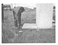
There are two side panels left which needs to be positioned onto the base slab. Place any of the side panels in the recess of the base panel (first 2 photos below), now push the bottom (1240) long rod through the panel and fasten with a M5 Nut (3rd photo below).
