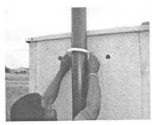
Once the vent pipe bracket bends have gone through the vent holes, push the vent pipe bracket with both your hands and hold on until the vent pipe bracket is fastened in the inside of the toilet, see photo below. To fasten the vent pipe bracket on the inside of the toilet structure, pull the two bends towards each other and fasten the bracket with the M6 x 50 gutter bolt and nut, see photos below.
