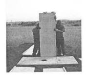
Place one back panel tightly next to the side panel (1st photo below), push the two 945 rods (2nd and  $3^{rd}$  photos) from the side of the side panel through the back panel to where the hole ends.
