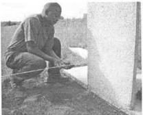
Place the 2<sup>nd</sup> back panel next to the first back panel, please remember to make sure the smooth side of the back panels are in the inside of the toilet structure, see photo below.
